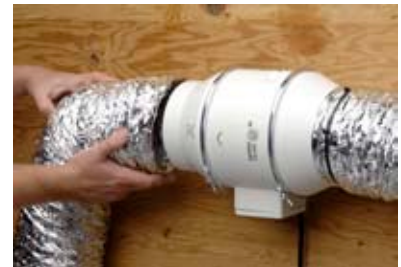
Connect the ducts.
